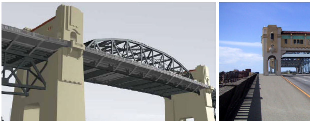
Figure E3 - Full-length outward sidewalk widening
