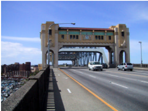
Figure E6 - Existing roadgate
