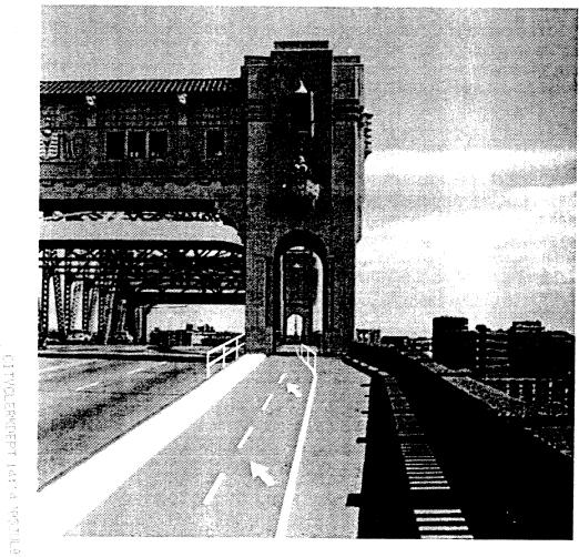
In contrast to a typical intersection, this treatment provides for a continuous flow of cycling and pedestrian traffic and physically separates user groups where a risk of conflict exists. The
