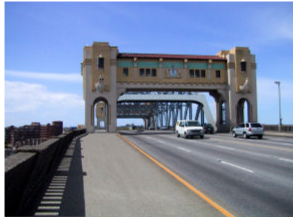
Figure 5 - Roadgate with sidewalk widening, except at towers
