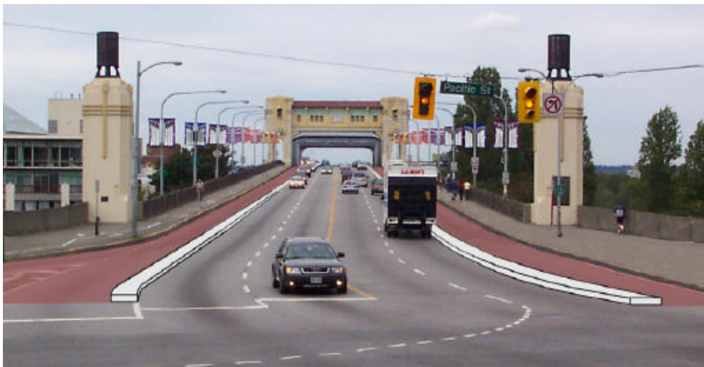
Figure F2 - Road-level bike lanes
