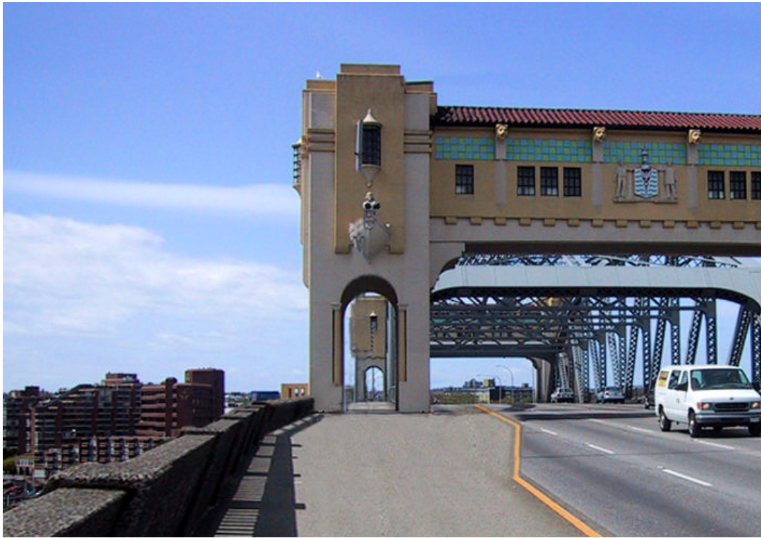
Figure F1 - Transition between 4-lane inward sidewalk widening and 6-lane outward sidewalk widening.
