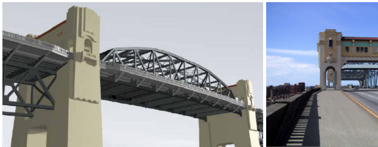
Figure E4 - Outward sidewalk widening, except at the towers (piers 3 & 4)
