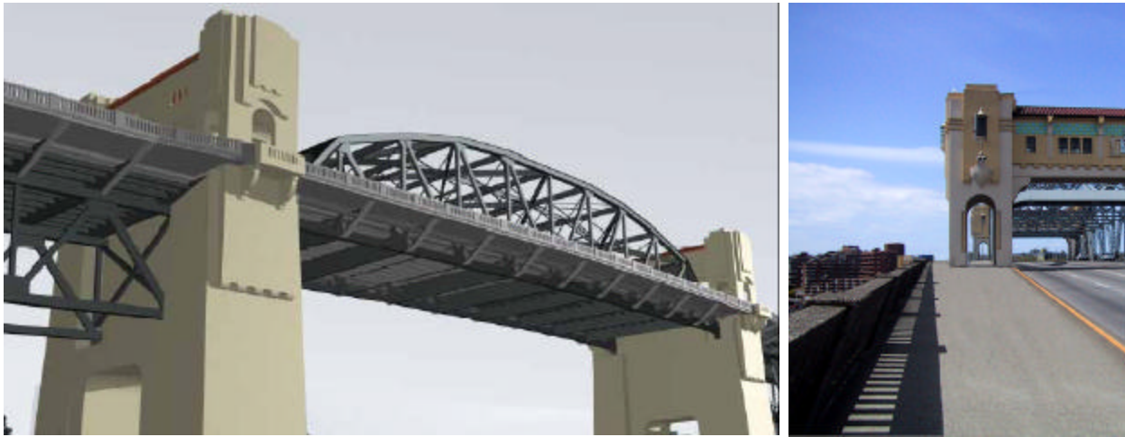
Figure E3 - Full-length outward sidewalk widening
