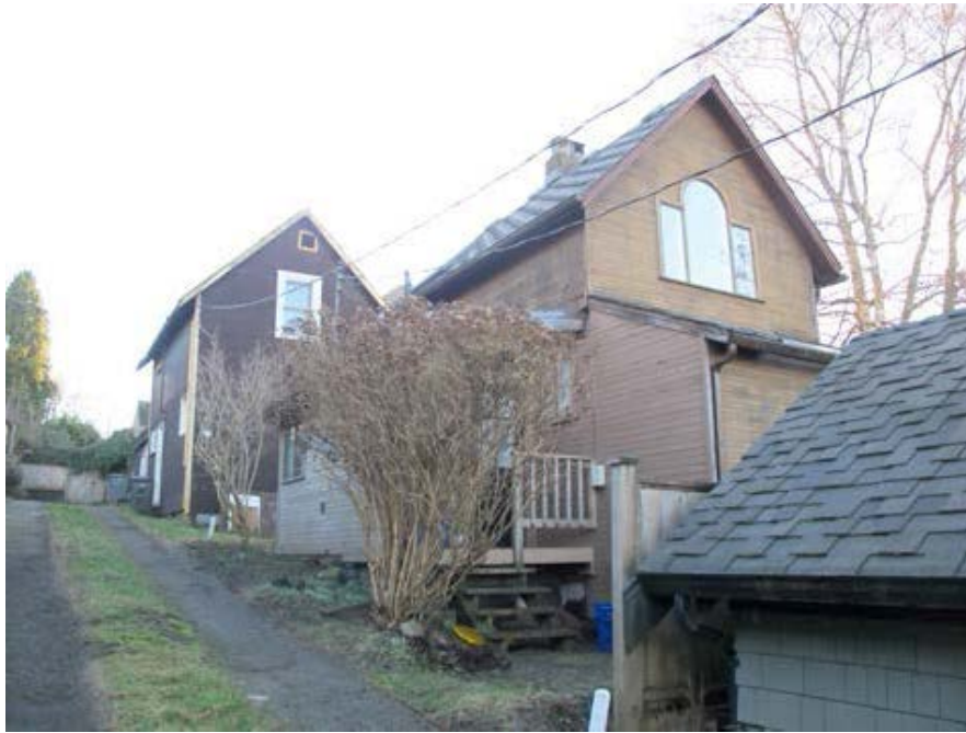
Photo 3: 1610 Stephens St. (Foreground) and 1618 Stephens St. (Background)
