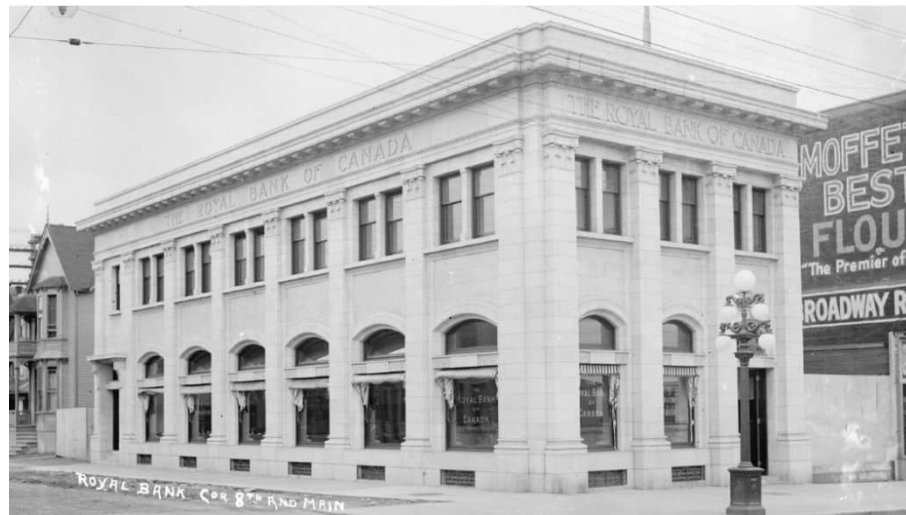
Figure 9: The Royal Bank of Canada Building, circa 1912, as viewed from the southeast corner of Main Street and East 8th Avenue
