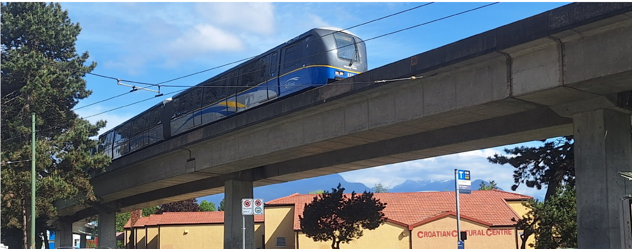
SkyTrain guideway near Commercial-Broadway station
