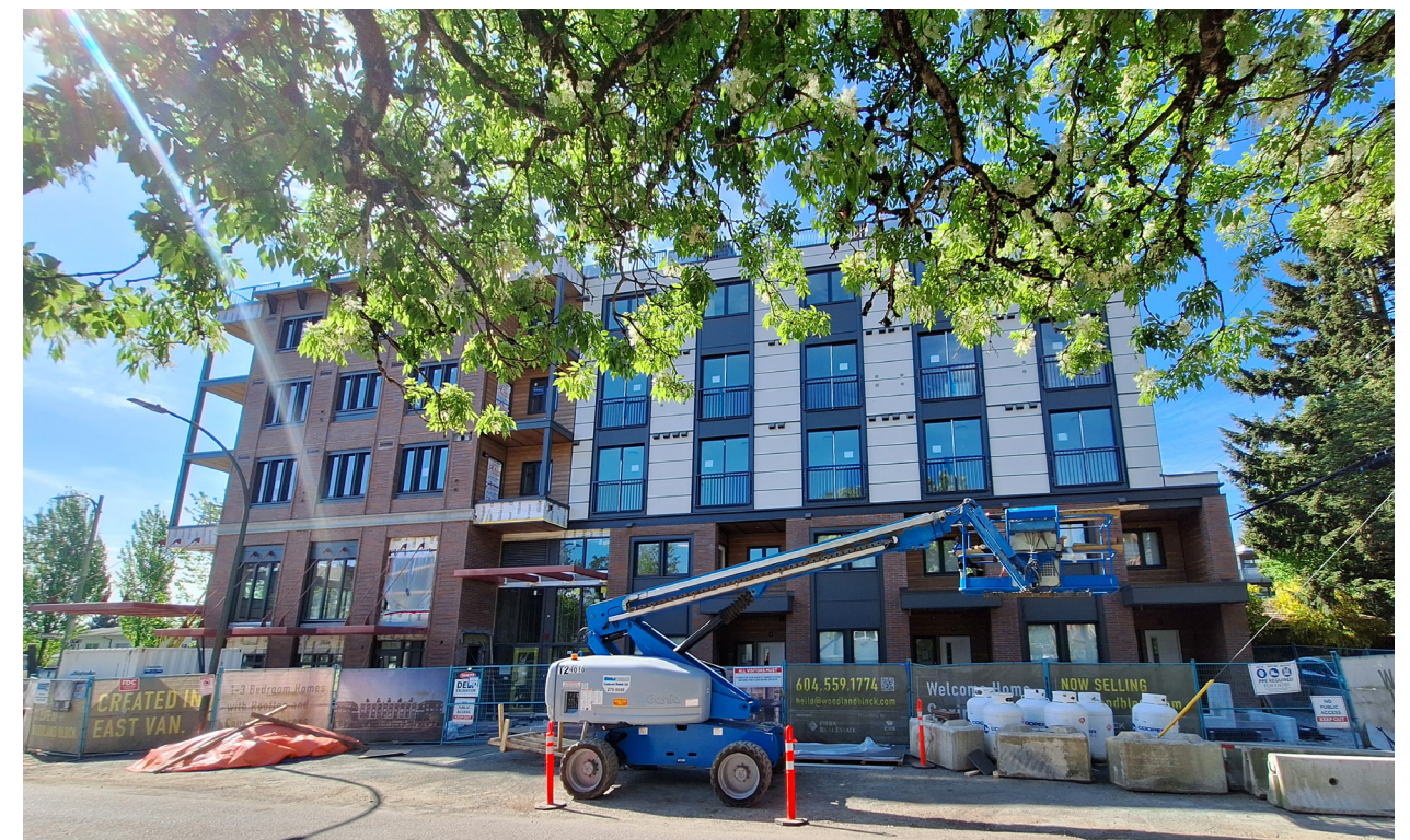
Construction site for a new mixed-use development
