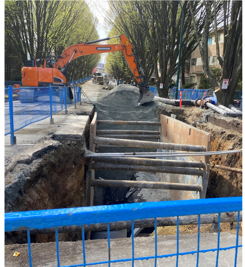
Oak St Sewer Separation Upgrade
