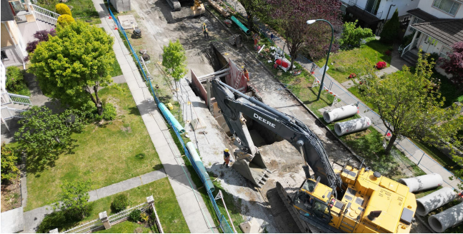
Sewer main replacement 25 km across Dunbar, Kerrisdale, Shaughnessy, Hastings-Sunrise & Kitsilano with est. completion in 2027, $226M
