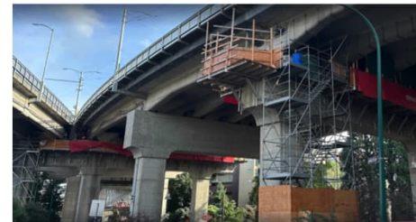
Granville/Cambie Bridge seismic upgrade/rehab › Cambie: Seismic upgrade along marine span and north approach, as part of Phase 2 › Granville: Phase 1 of South Approach repairs, Phase 2 of Coating Renewal at north end
