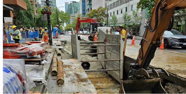
Water main renewals Replace 1 km transmission main (Pender) + 40 km distribution mains in various locations by 2027, $100M
