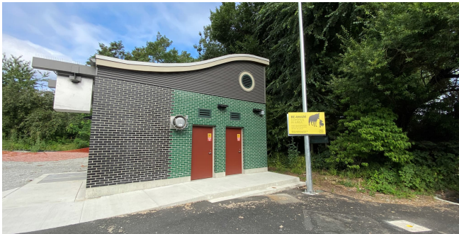
Renewal and upgrades of 4 pump stations Renew/upgrade 4 pump stations: Raymur (complete), Dunbar (by 2026), Thornton (by 2027), Terminal (by 2028), $30M
