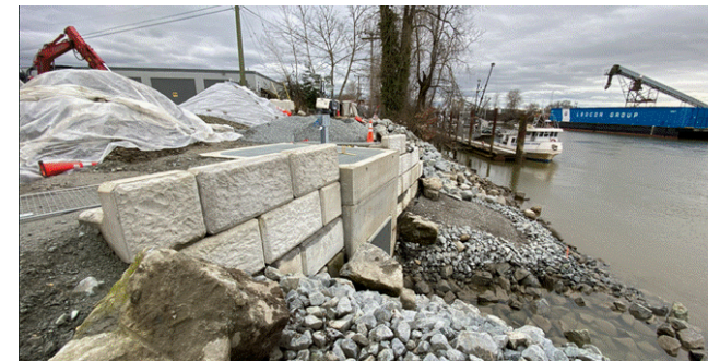
Outfall and flood management upgrades Replacement or upgrade of three outfalls, 3 km of coastal flood management and 0.5 km of creek/ditch flood management, $22M
