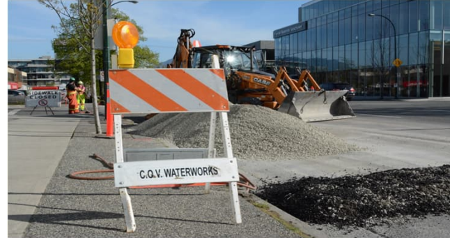
Water main renewal and replacement of 3 km of transmission mains (Arbutus, W 37th, Charles) and 40 km distribution mains throughout the City, $145M
