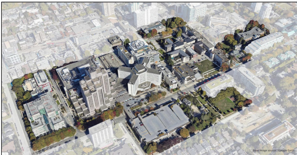
Figure 3: Aerial view of VGH Campus consisting of the VCH owned lands.
