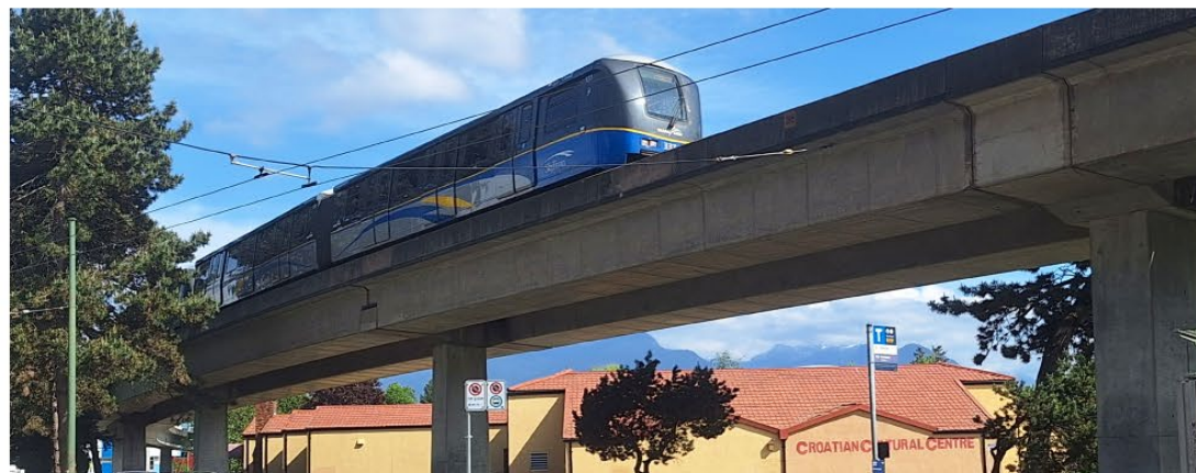
SkyTrain guideway near Commercial-Broadway station
