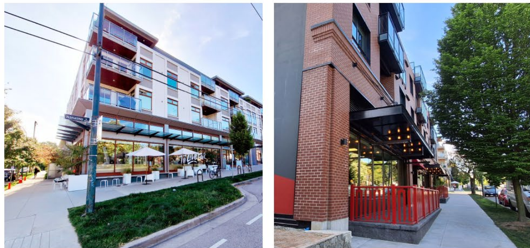
Street widening and patios from recent development of mixed-use buildings along Nanaimo Street
