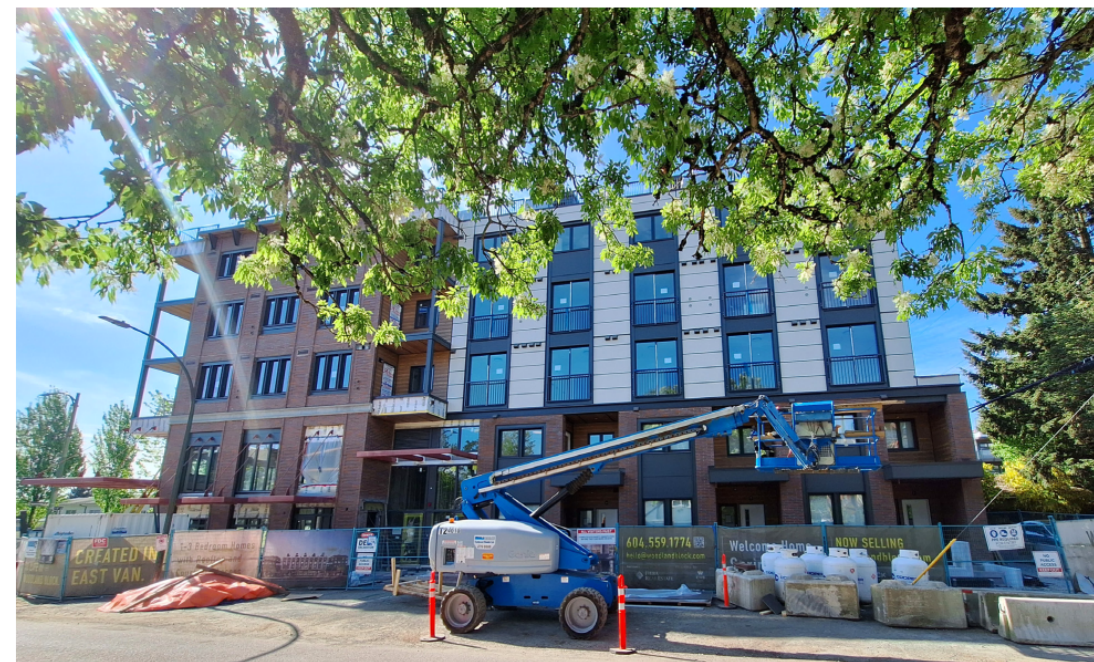
Construction site for a new mixed-use development
