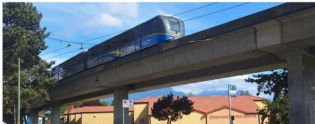
SkyTrain guideway near Commercial-Broadway station
