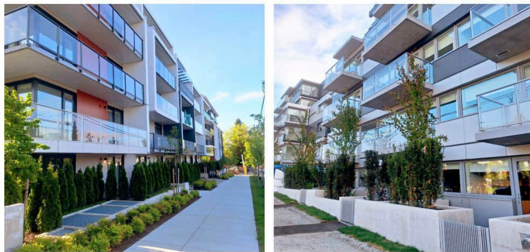
Recently built 6-storey residential developments along Oak Street
