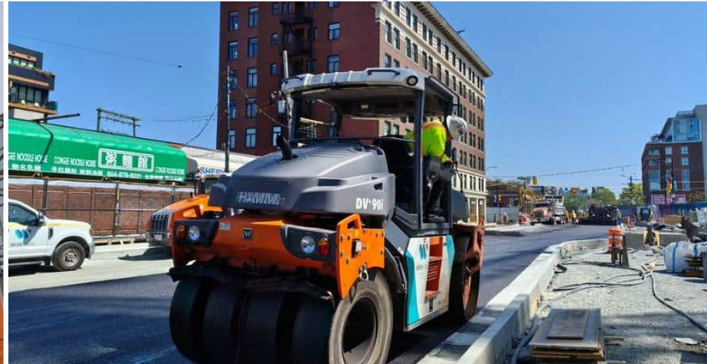
Traffic deck removal and street reconstruction underway
