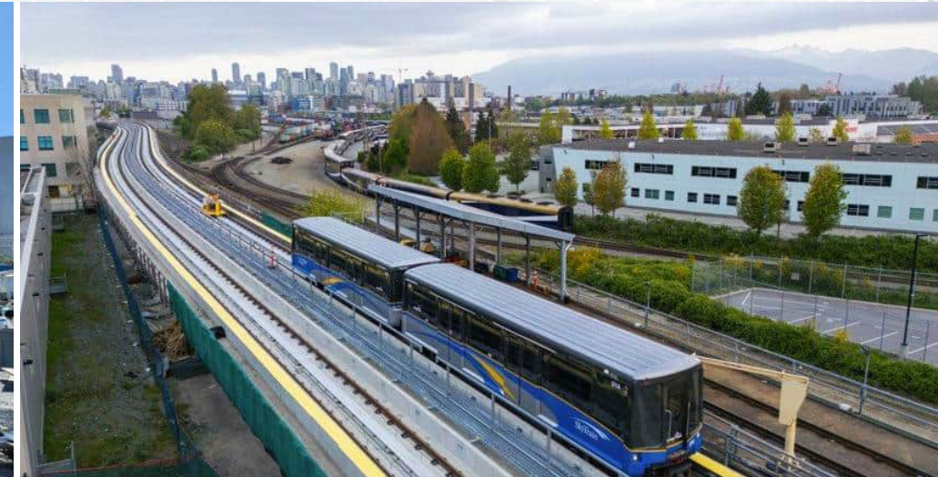
Trains ready for testing on elevated guideway
