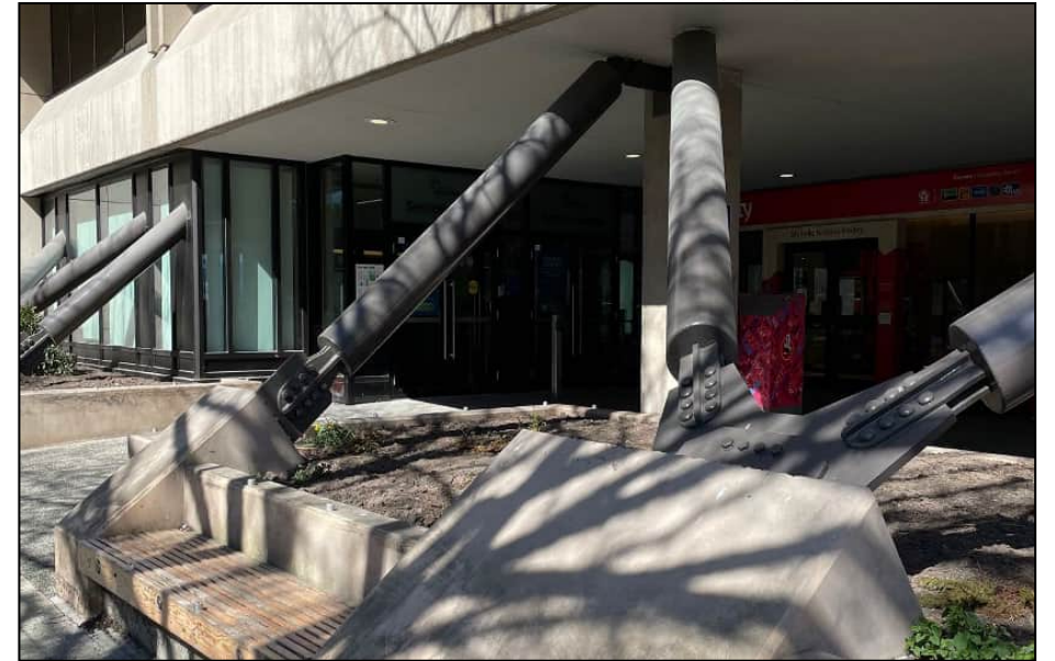
Upgrade elements from the seismic retrofit of 515 W. Tenth Street
