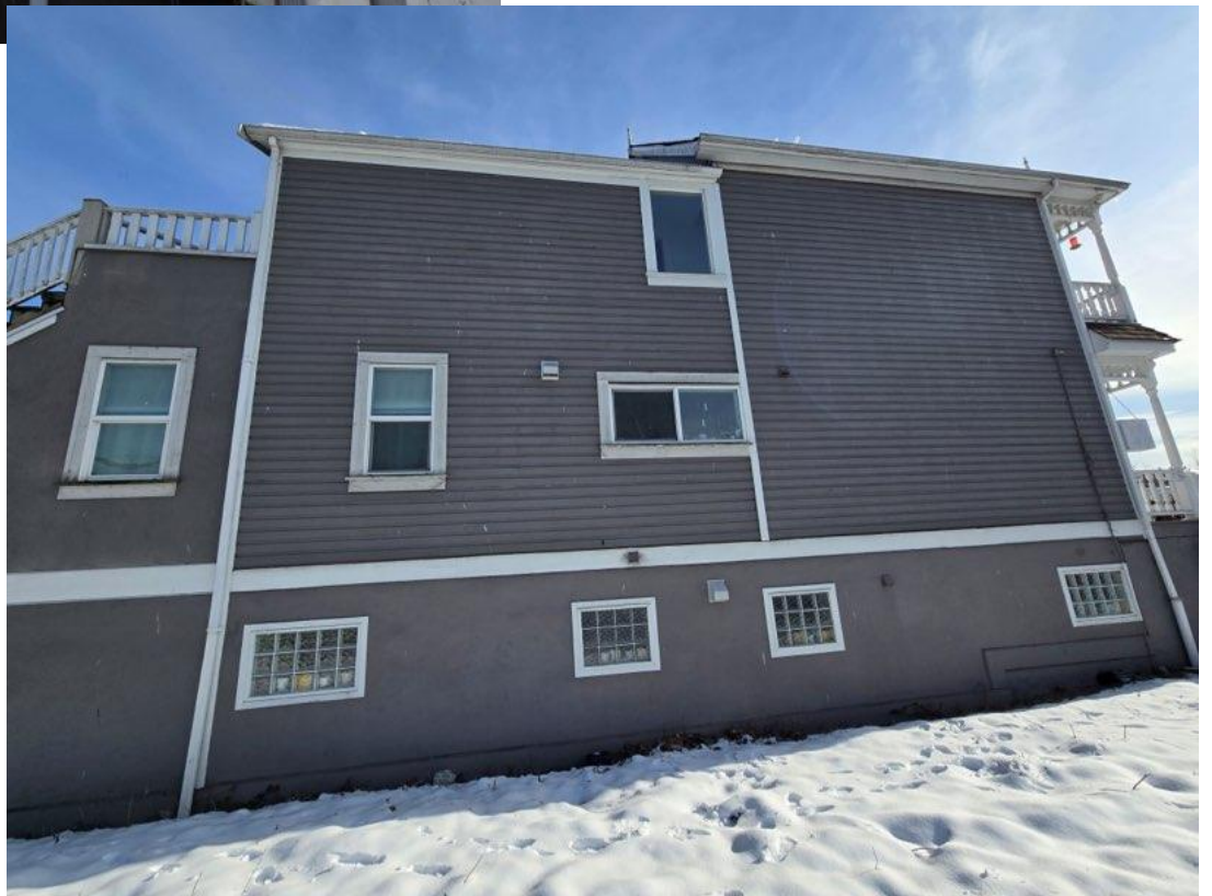
Side view (west elevation)
