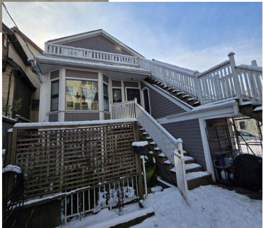
Rear view (north elevation)
