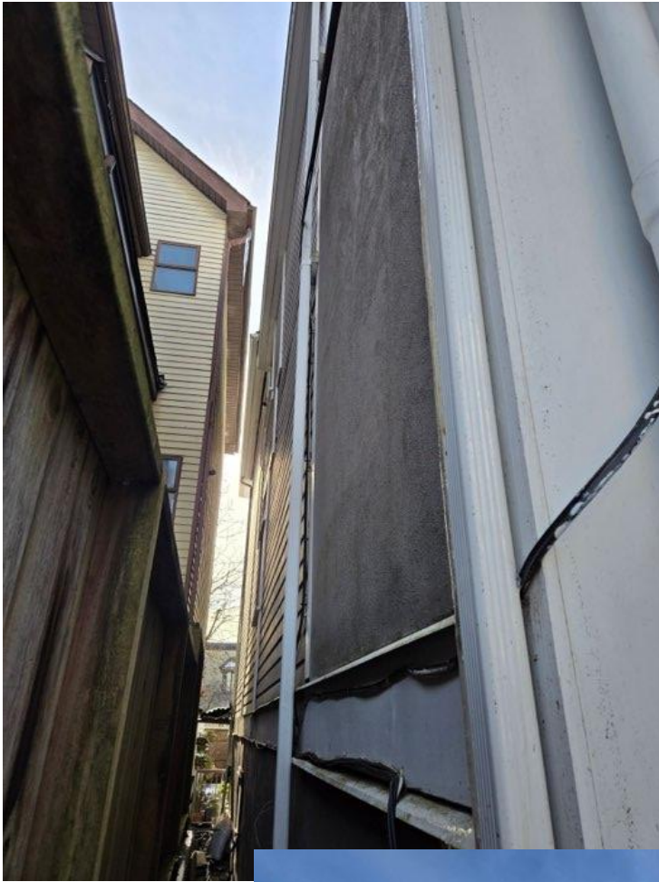
Side view (east elevation)
