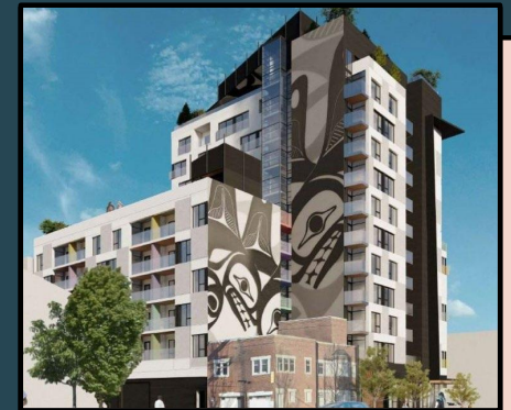
In progress - 172-unit social housing development at 401 Jackson – Aboriginal Land Trust – this is a family and senior focused development
