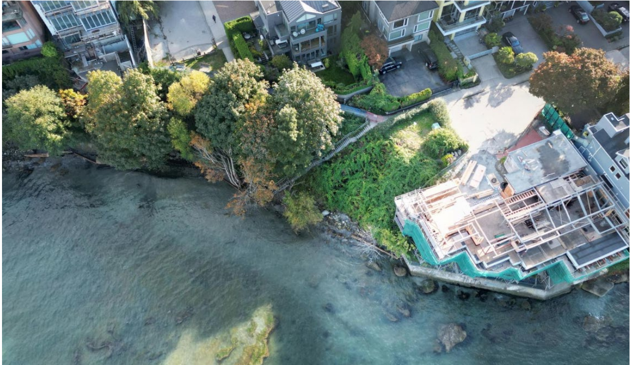
Figure 3: Overview of beach access.
