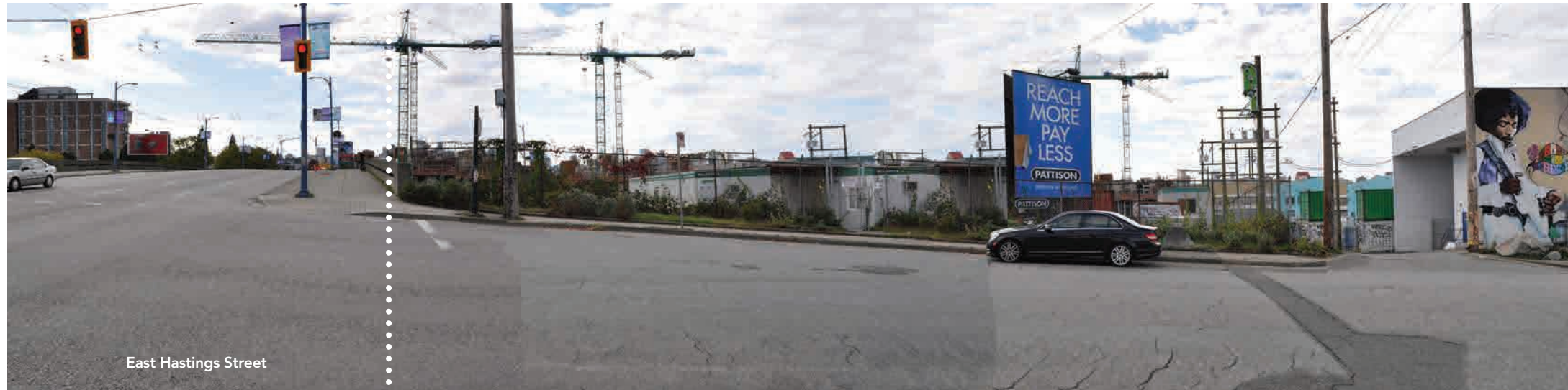
D Glen Drive Looking West
