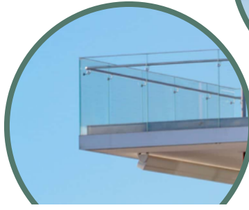
METAL AND GLASS BALCONY GUARD
