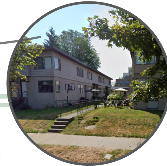
EXISTING MIDBLOCK CONNECTOR ON SITE FROM W 3RD TO LANE (WHOLE FOODS)
