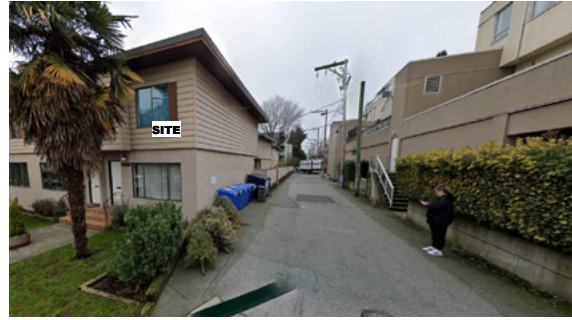
SW LANE VIEW FROM VINE ST
