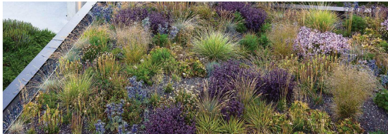
GREEN ROOF PLANTING WITH GRASSES, SEDUM, PERENNIALS
