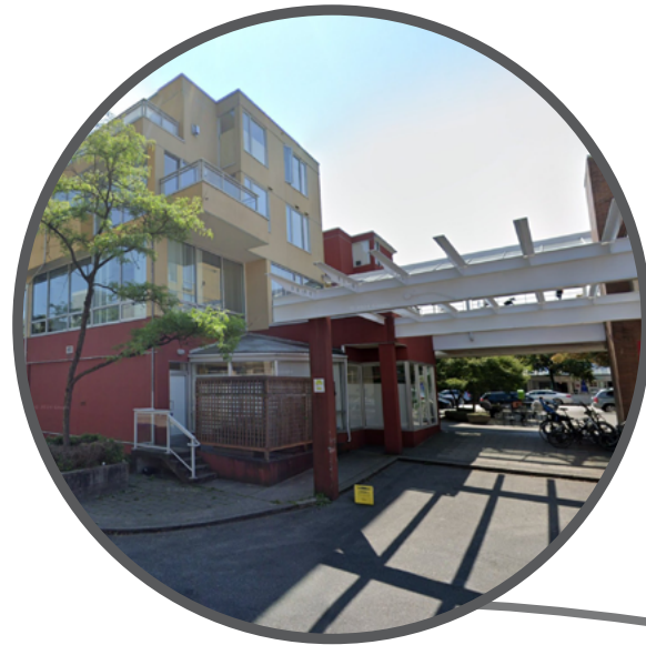
EXISTING MIDBLOCK CONNECTOR FROM LANE TO W 4TH
