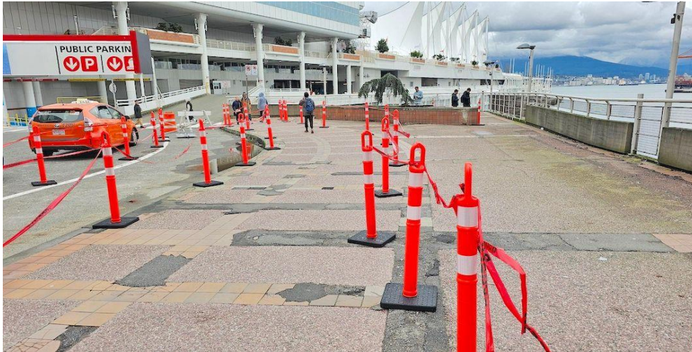
Canada Place (Howe St, W Cordova to Canada Pl) sidewalk renewal - 2024
