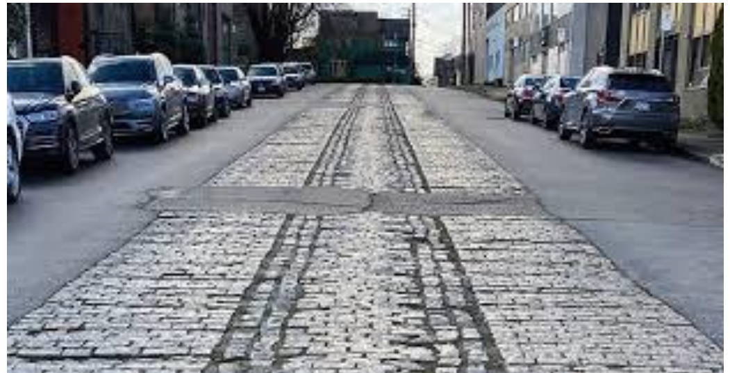
Granite pavers on Frances St (Clark to Vernon)
