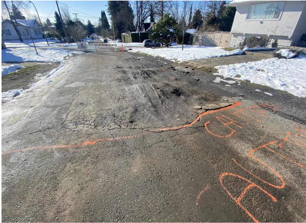
Example of freeze/thaw damage to road Hudson St (W 57 th to W 58 th Ave)
