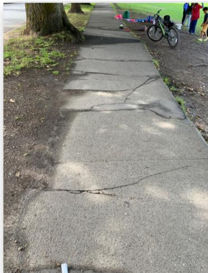
2600 Vine St - west side (adjacent to Connaught Park)
