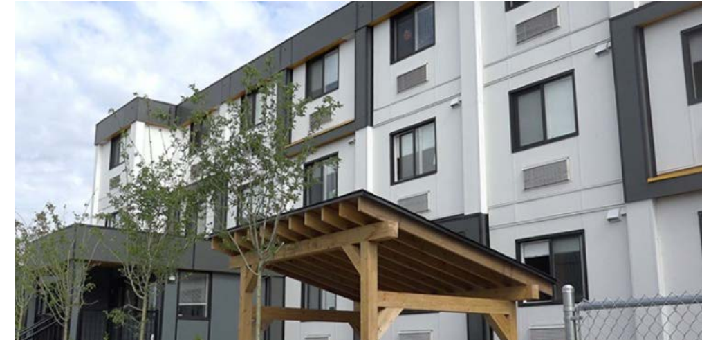
Temporary Modular Housing: 2131 Franklin St.
