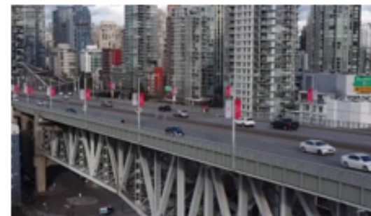
Cambie Bridge rehabilitation & seismic upgrades ($12M)
