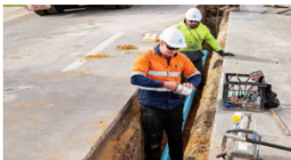
Distribution Main Renewal ($24M)
