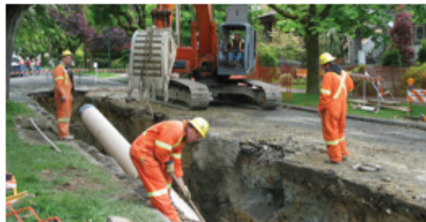
Sewer Main Renewal ($45M)
