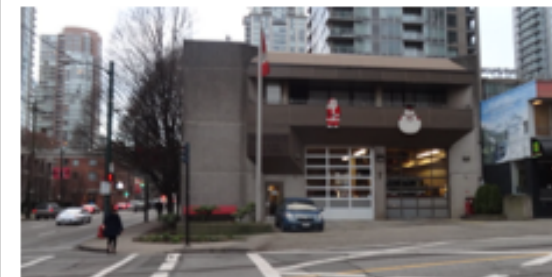
Renewal and Expansion of Downtown South firehall ($13M)
