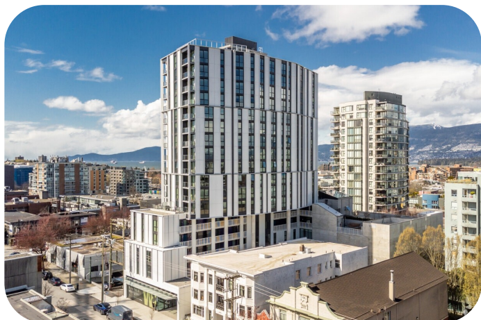
Social Housing - Vancouver Masonic Centre
