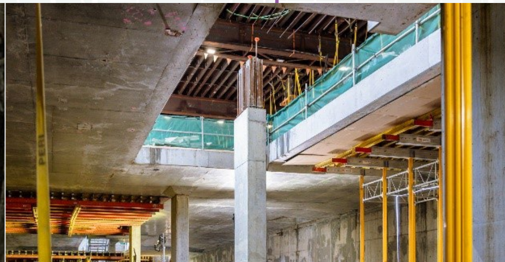
Traffic decking at station areas complete
