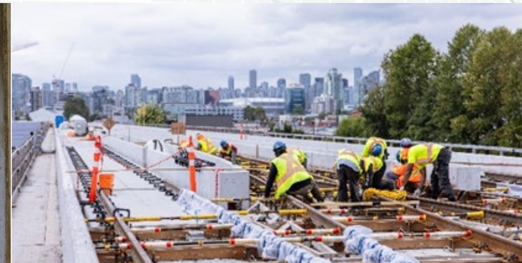
Elevated guideway begun rail installation
