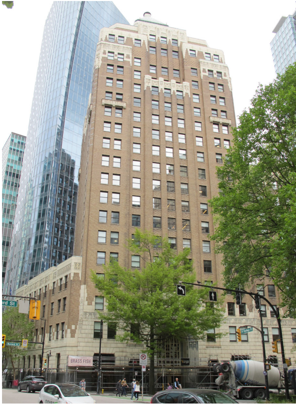
Single assembly one-over-one hung windows of the Marine Building present on floors above the ground floor, 2024. (DLA)
