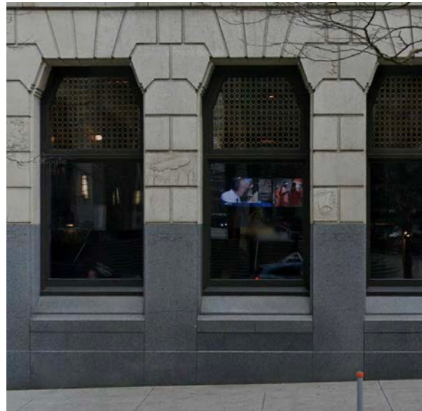
Example of tapered window openings and windows of ground floor, 2022. (Google)
