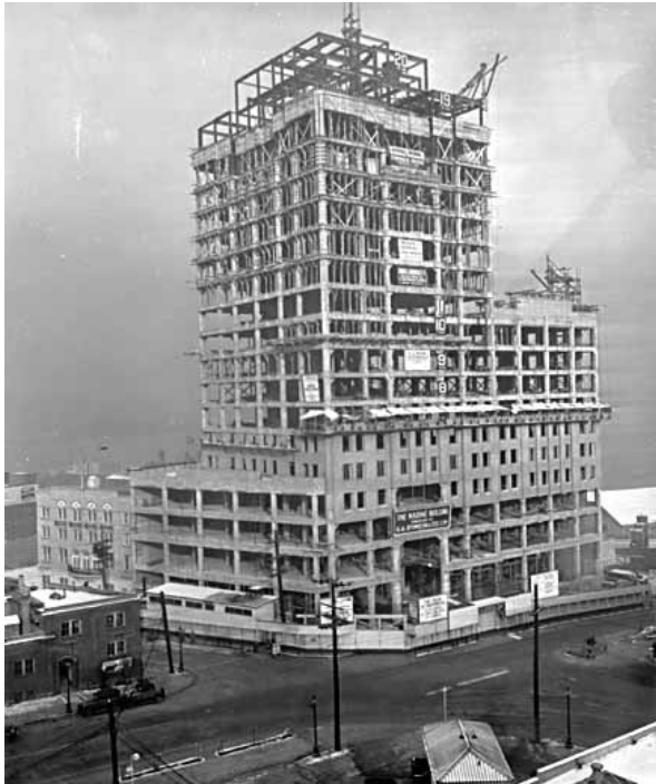
Structure of the Marine Building under construction with installation of brick on lower floors of the tower underway, 1929. (VPL 11994)
