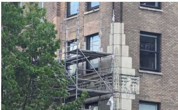
Left Top and Bottom: Completed mock up using salvaged and new brick viewed from scaffolding and street level. Visual difference between the new brick and the existing is significant and closer colour matched brick should be considered, 2024. (RJC, DLA) Right: Example of Vancouver building where shelf angles were replaced. Note banding evident in brick where shelf angles were replaced, 2024. (DLA)
