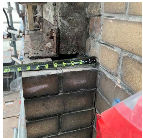
Top and Bottom: Condition of brick showing cracks at mortar joints and through brick, and past repointing work. Corroded condition of existing shelf angle and lack of shelf angle on return shown, 2024. (RJC)
