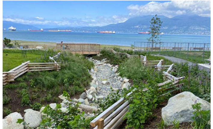
Above: Completed restoration works at Tatlow Creek.
