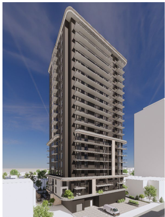
Building view from North East
