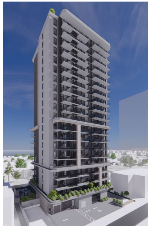
Building view from North East
