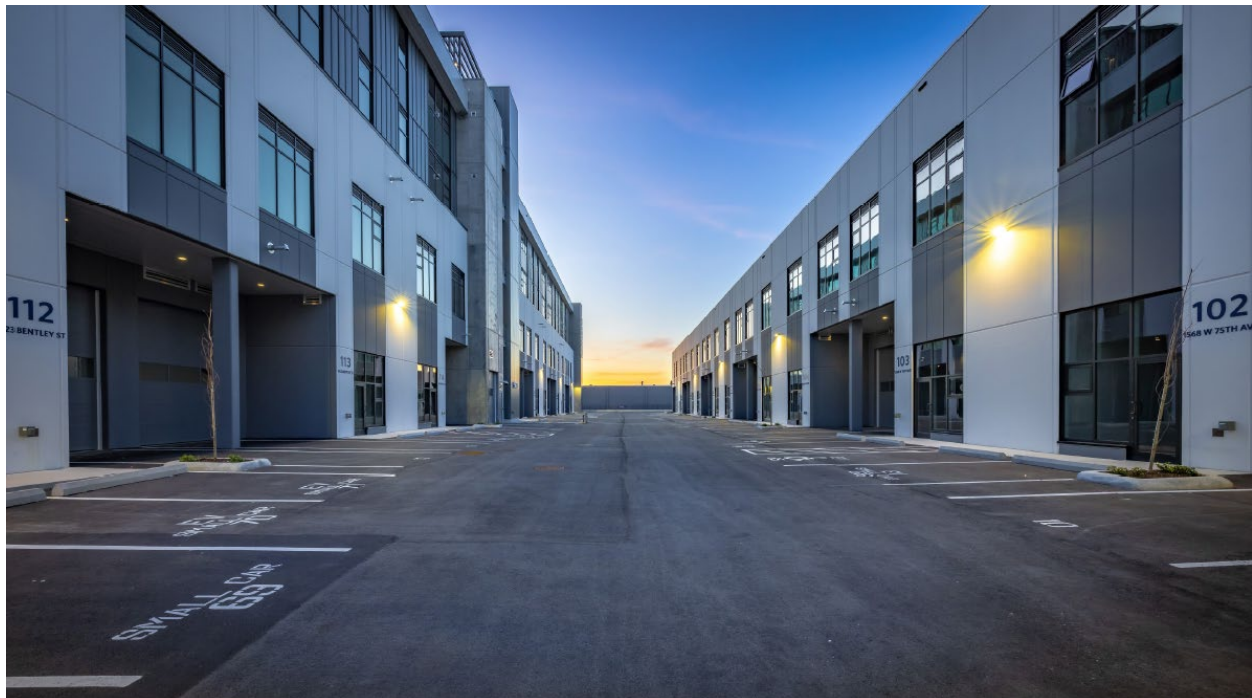
Figure 3: South building at left and north building at right as seen from central mews
