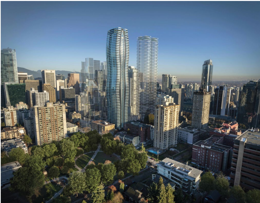
Figure 3: Proposed Building Looking Northeast
