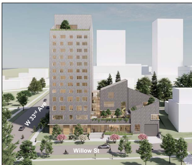
Figure 2: View of the Building, Looking East
