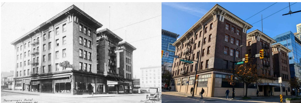
Figure 1, Original building circa 1910, photo left. Building at time of this report, photo right.
