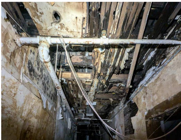
Figure 9, Top floor ceiling, south end hallway.
