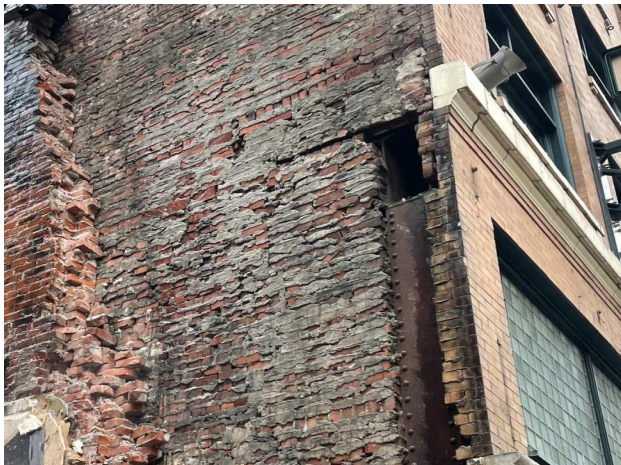
Figure 35, Example of steel beam/column support.
