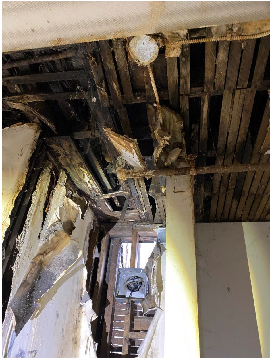
Typical Condition below SE skylight
