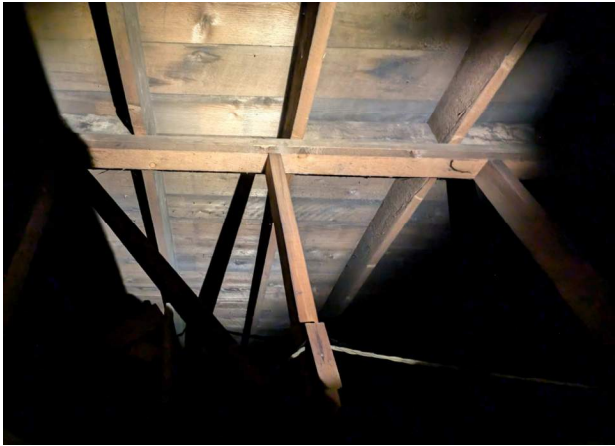
Figure 3, Roof rafters on pony walls.
