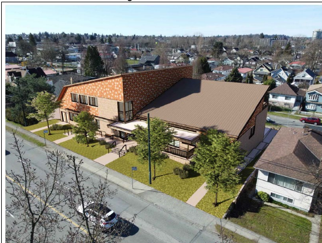
LOOKING SOUTHWEST ON VICTORIA DRIVE
