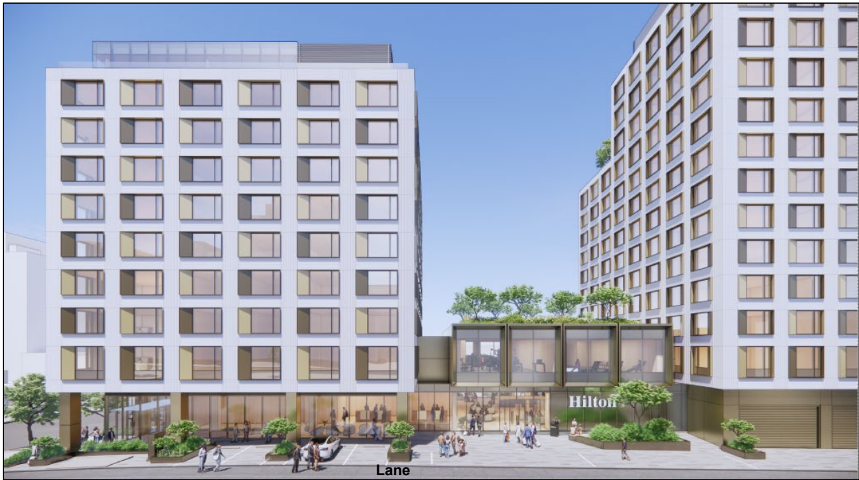
View from Lane Looking North
