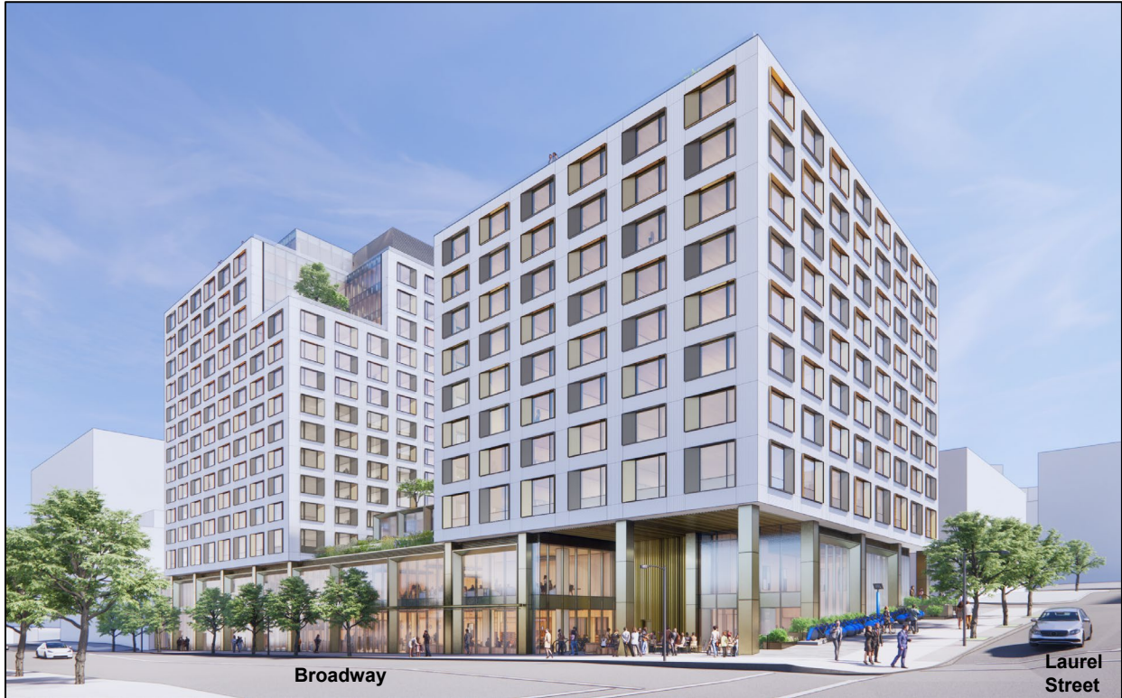
View from Broadway and Laurel Street Looking Southeast
