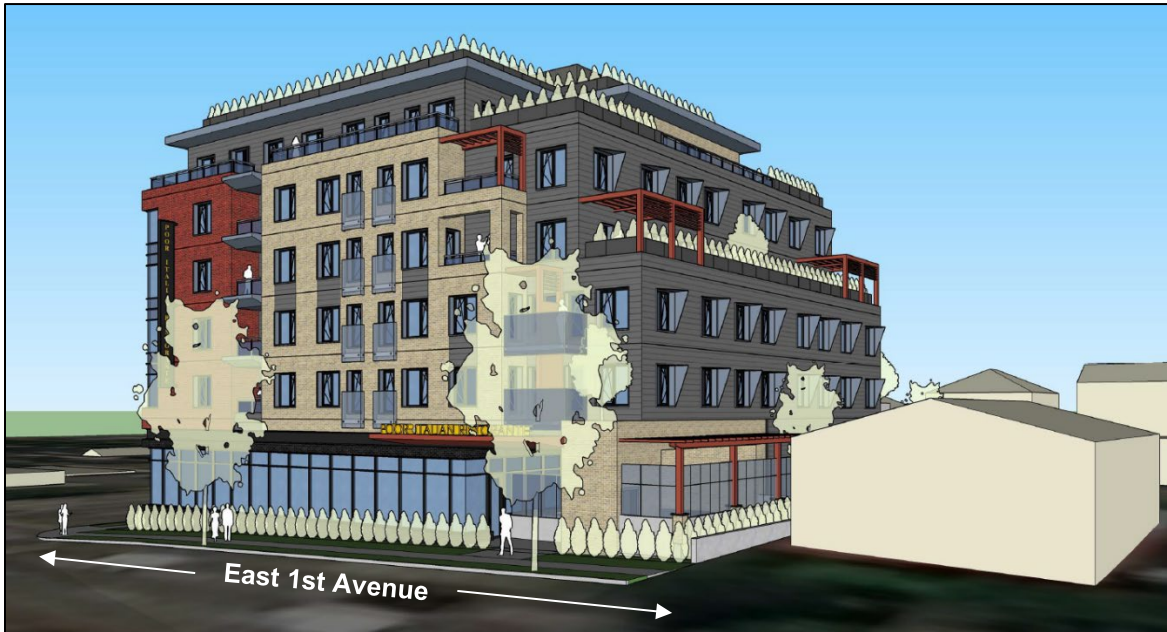
Figure 3: Perspective from East 1st Avenue Looking Southeast
