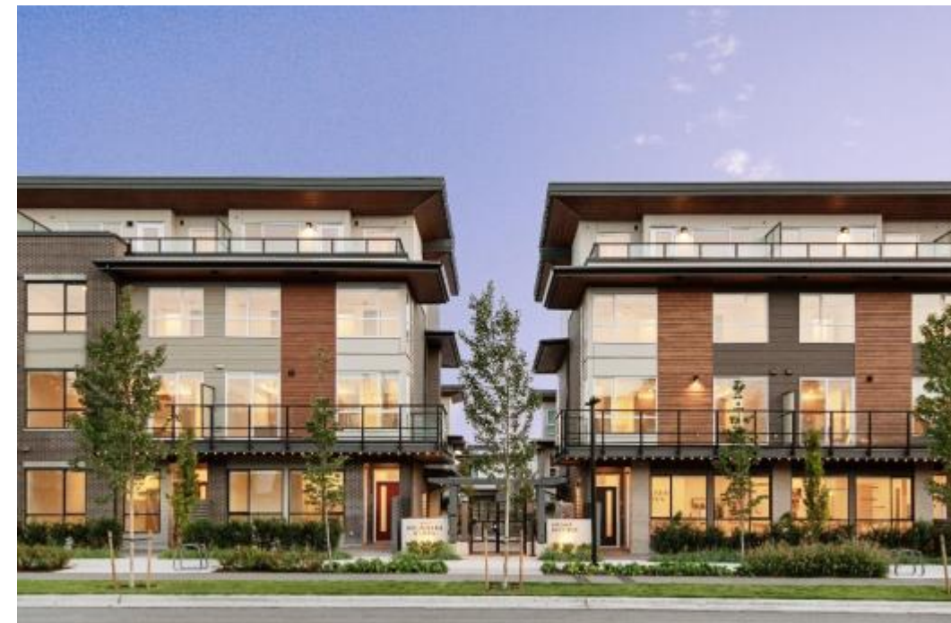
Founders Block North & South, North Vancouver
