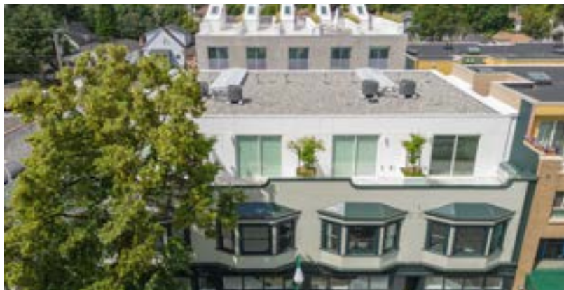
Broadhurst and Whittaker Block (Francis Lai Photography)
