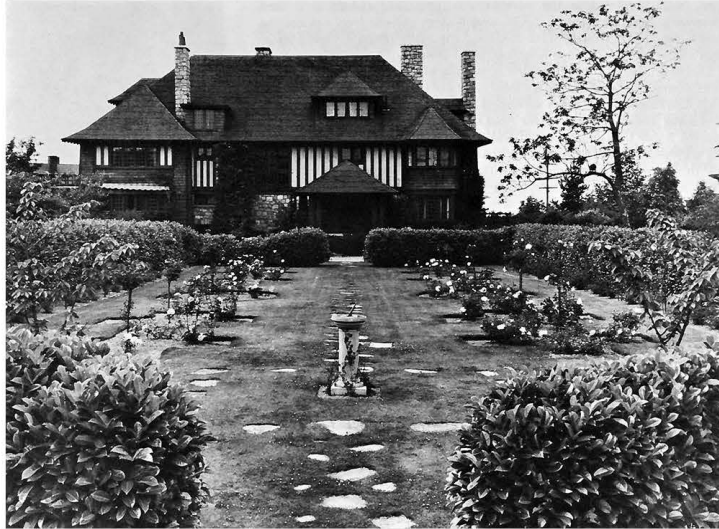
Figure 3 The Nichol House [W.J. Moore, photographer. City of Vancouver Archives Bu P567]. The house design exhibits a tripartite composition with the display of a discernible base, middle and top. The significant front yard rose garden, a protected heritage feature, is an integral component of the heritage value of this property.
