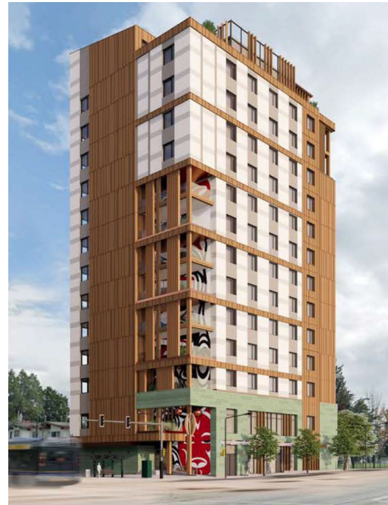
406-1410 E King Edward Ave 109 permanent supportive units under construction.
