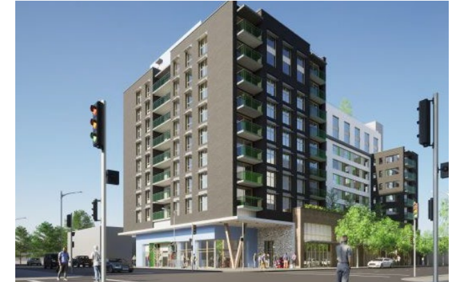
525 Powell St 158 social units under construction with ground floor retail.
