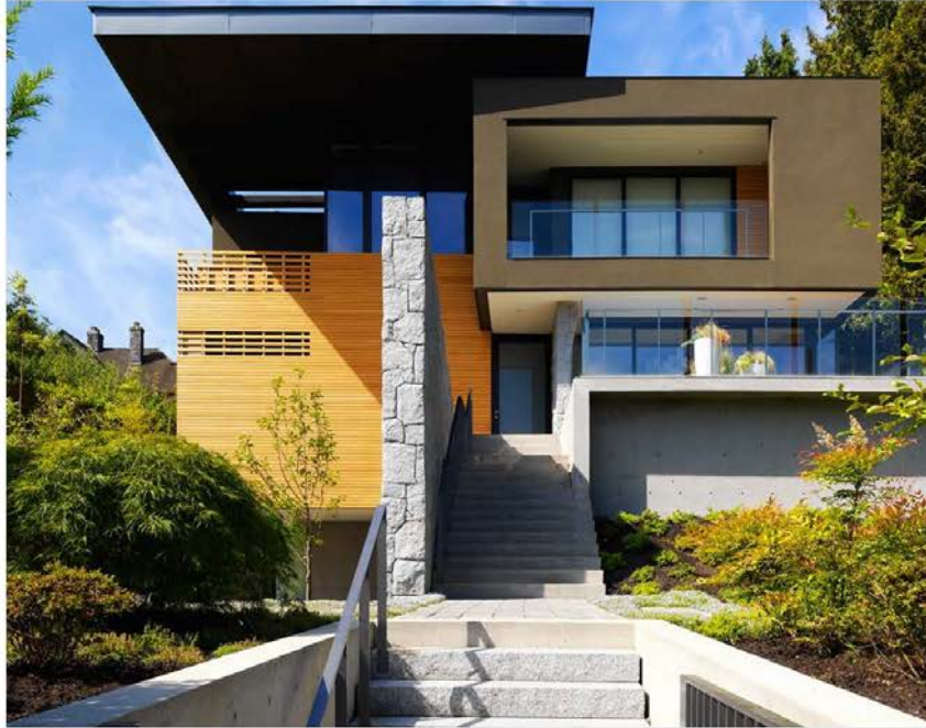
Figure 7 1098 Wolfe Avenue, photo courtesy of Measured Architecture, 2014. Contemporary expression in conjunction with a carefully crafted landscape design
