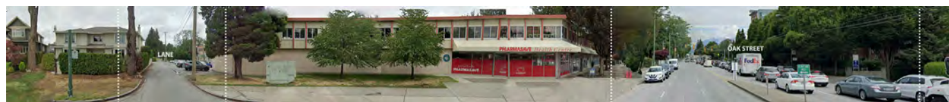
W 42ND AVENUE: NORTH VIEW, OAK STREET TO LANE
