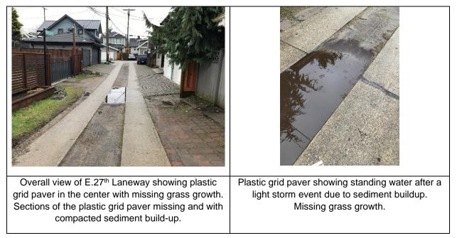
Maple St Laneway: Plastic grid paver (product: Golpla) is in poor condition with certain sections breaking apart and some missing leading to potholes. Gravel from the driving strips is mostly eroded. No grass growth with build-up of compacted sediment. Standing water observed in various pockets of the plastic grid paver.
