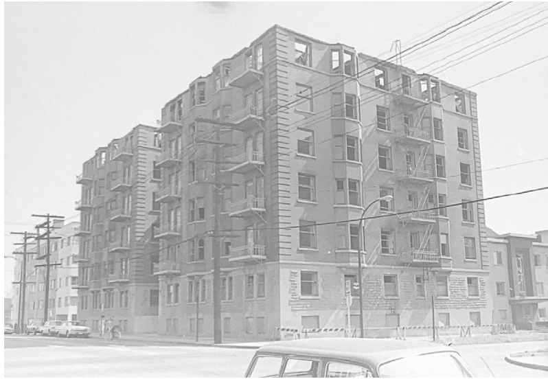
Damaged Building in 1966
