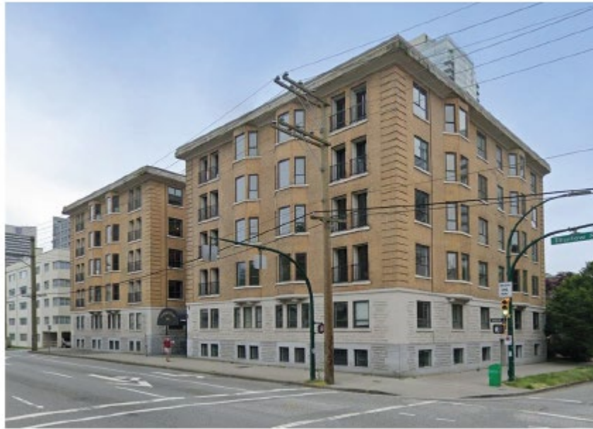
Current Existing Building 5 Storeys + Basement
