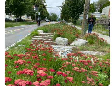
▼ Rain garden and bioswale at Woodland Drive and 2nd Ave (Source: City of Vancouver)
