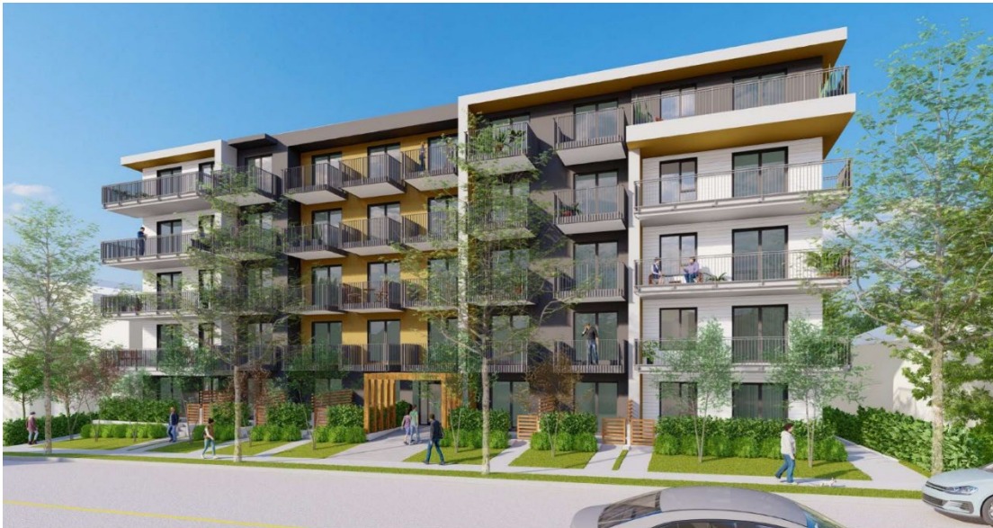
Figure 2: View of Proposed Development from 33rd Avenue (looking north)
