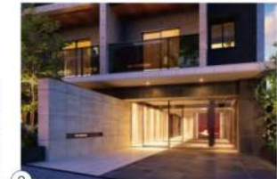
② Decorative Entrance Paving
