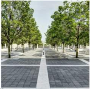
④ Decorative Paving Patterns with Concrete Banding
