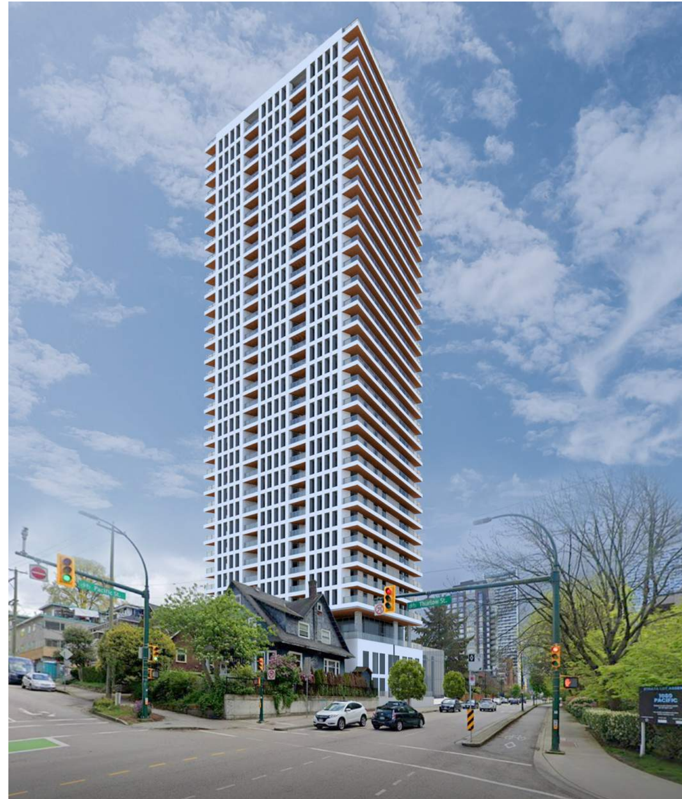
VIEW FROM INTERSECTION OF PACIFIC AND THURLOW STREETS - LOOKING EAST
