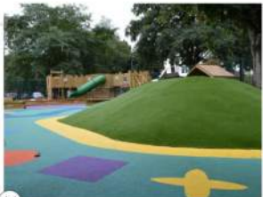
11 Outdoor Play Area with Turf Mound and Poured in Place Rubber
