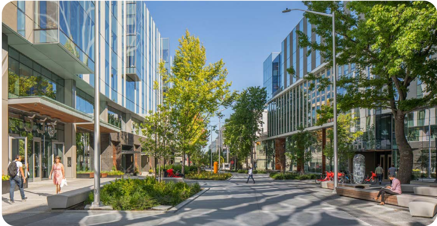
A pedestrian-oriented open space that balances circulation, green space and public amenity.
