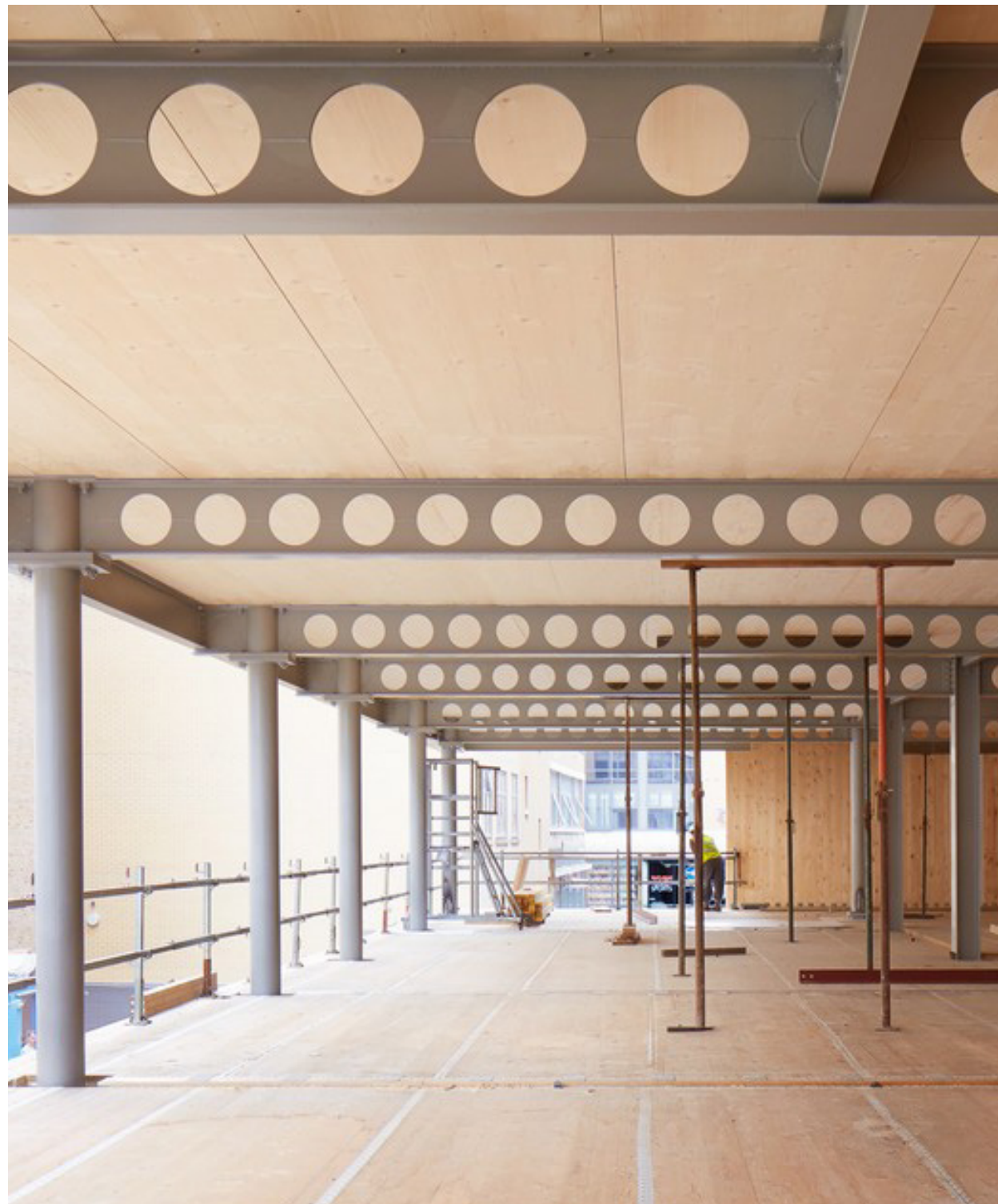
Curtain Place, Hybrid Mass Timber Building, London
