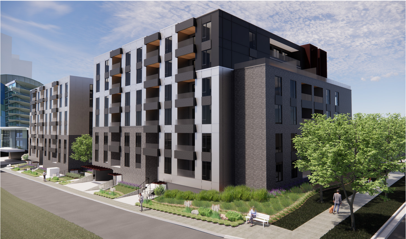
VIEW FROM REAR LANE AND W 65TH AVE
