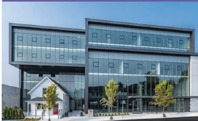
3.0 FSR | Manufacturing, Office, Restaurant
