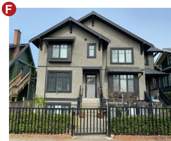
< 315-319 W16TH AVE (2014) Four-plex development, 3 storey with half sunken ground level. Ground units feature full height glazing and light wells.
