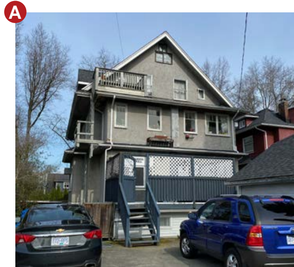
< 356 W15TH AVE (Built 1910, renovated in 1965) Four storey expressed as 2.5 storey. Character-defining elements include front and back gabled roof, dormers, and half-sunken garden level.
