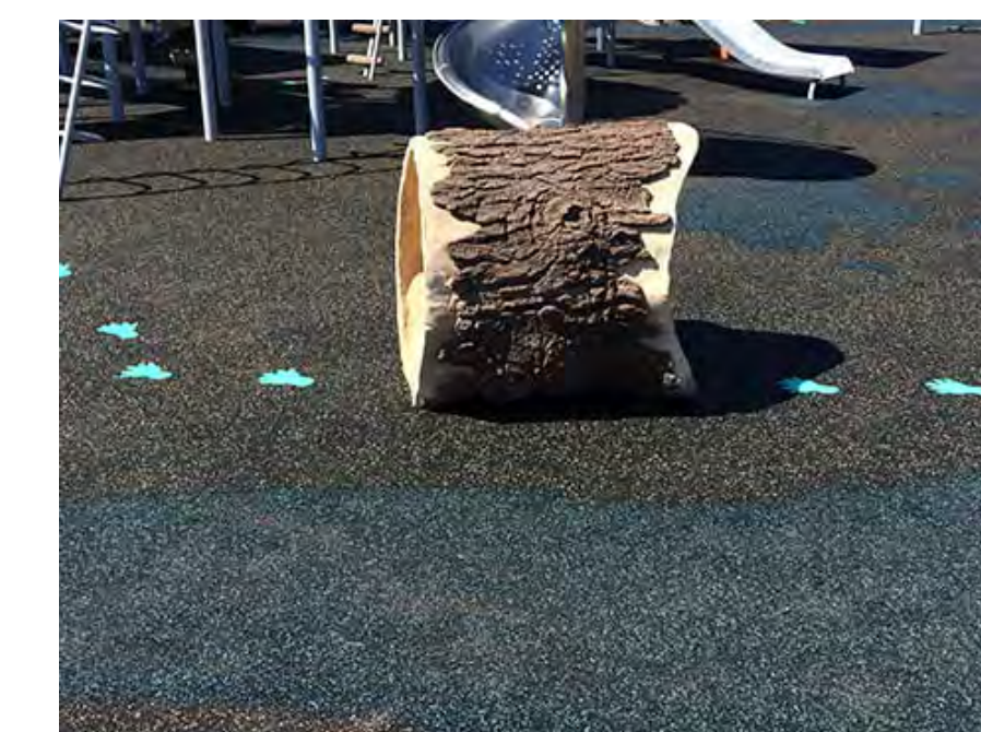
Example of resilient surface
