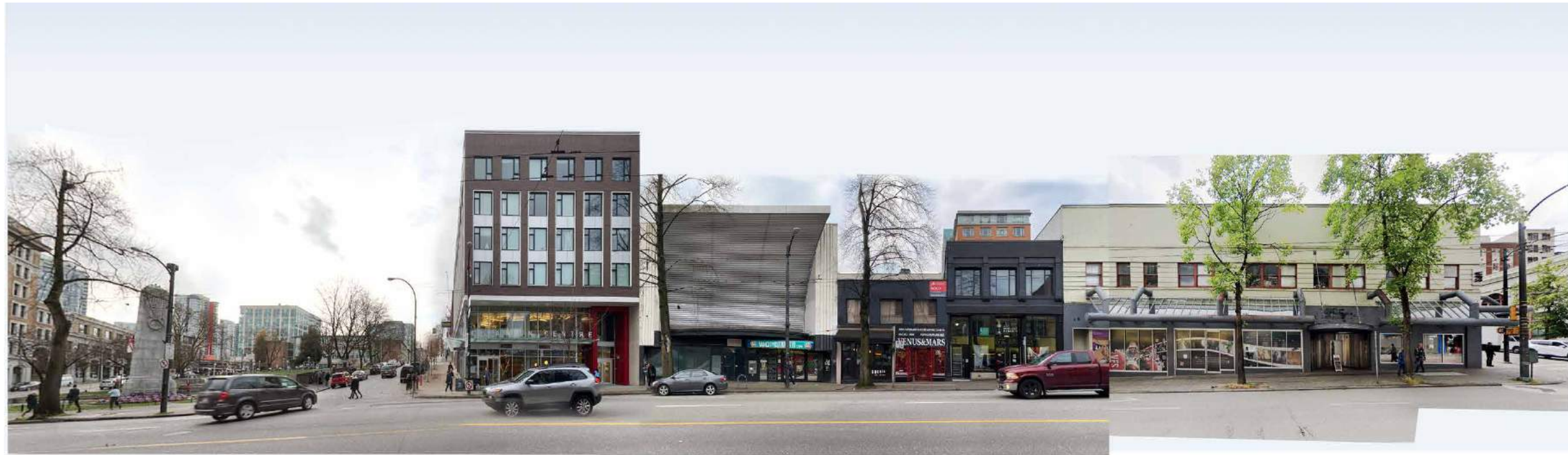
EXISTING STREETSCAPE ALONG WEST HASTINGS STREET
